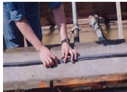
Connect two pieces by end-but joining
