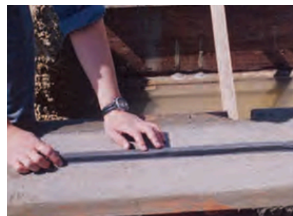
Place KuniSeal on joint and press in place
