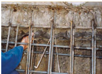
Slowly press on to connecting slab joint
