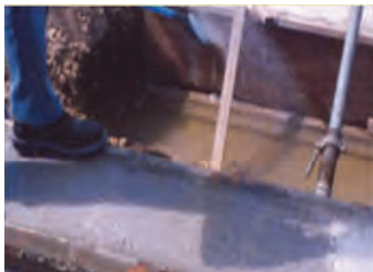
Brush off dirt and wet concrete joint
